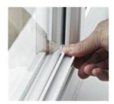
Place the top rail on the upper left corner of the window and slip it between the glass and the rubber gasket by pushing firmly, then slide the other end of the tab in the upper right corner of the window, as illustrated in the image above.
