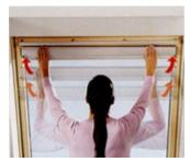
Fit the aluminium side rails to the frame of the window.
